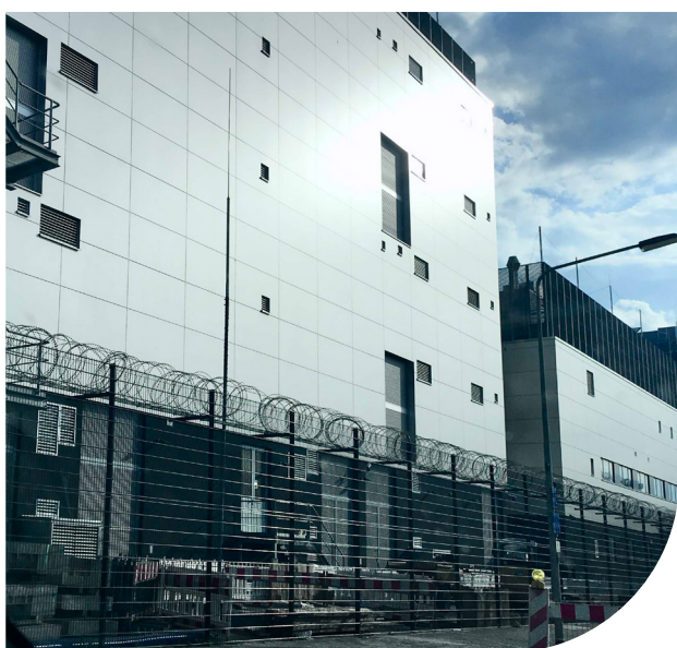
EXA Infrastructure data center, Frankfurt, Germany. Photo by KaiKemmann/Wikimedia Commons.
