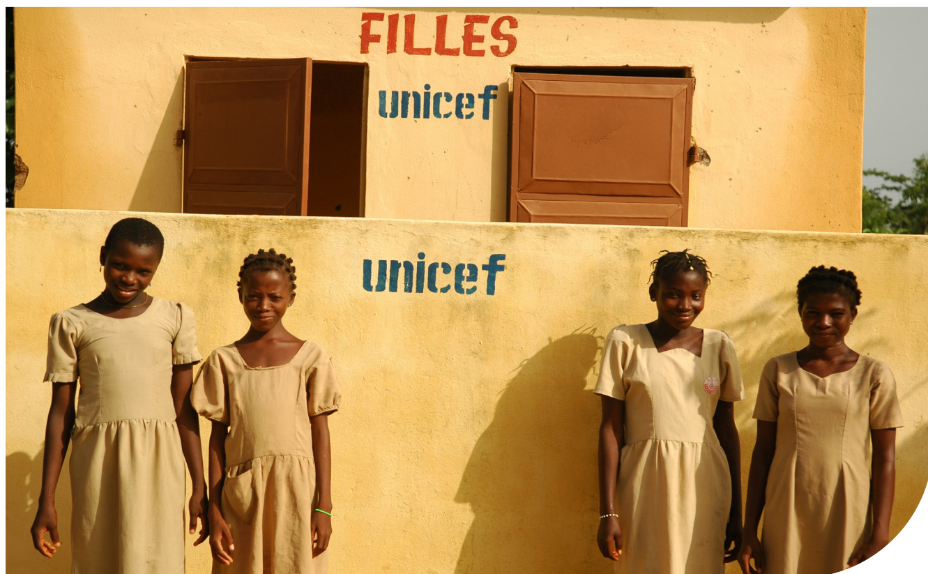
Schoolgirls stand outside a newly built girls' toilet block at their school in Togo, where poor sanitation remains a major health risk for children and communities.
