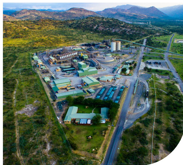
Two Rivers platinum mine, South Africa. Photo by Ryanj93/Wikimedia Commons.
