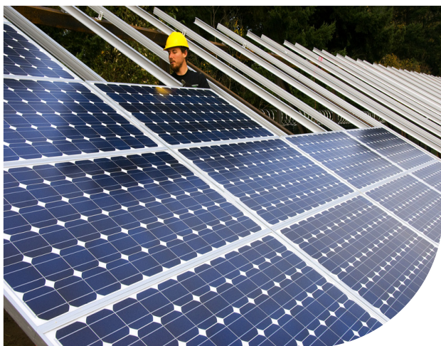
Workers installing solar panels. These panels incorporate critical minerals. Photo by Oregon Department of Transportation.
