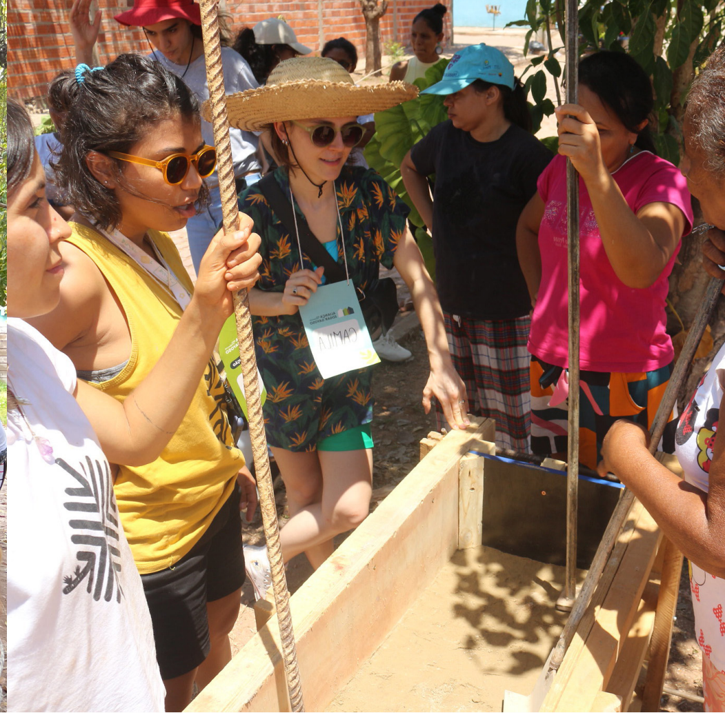
Teresina, Brazil: Earth construction workshop at Residencial Edgar Gayoso, October 2023. © Eduardo Sousah / WRI Brasil
