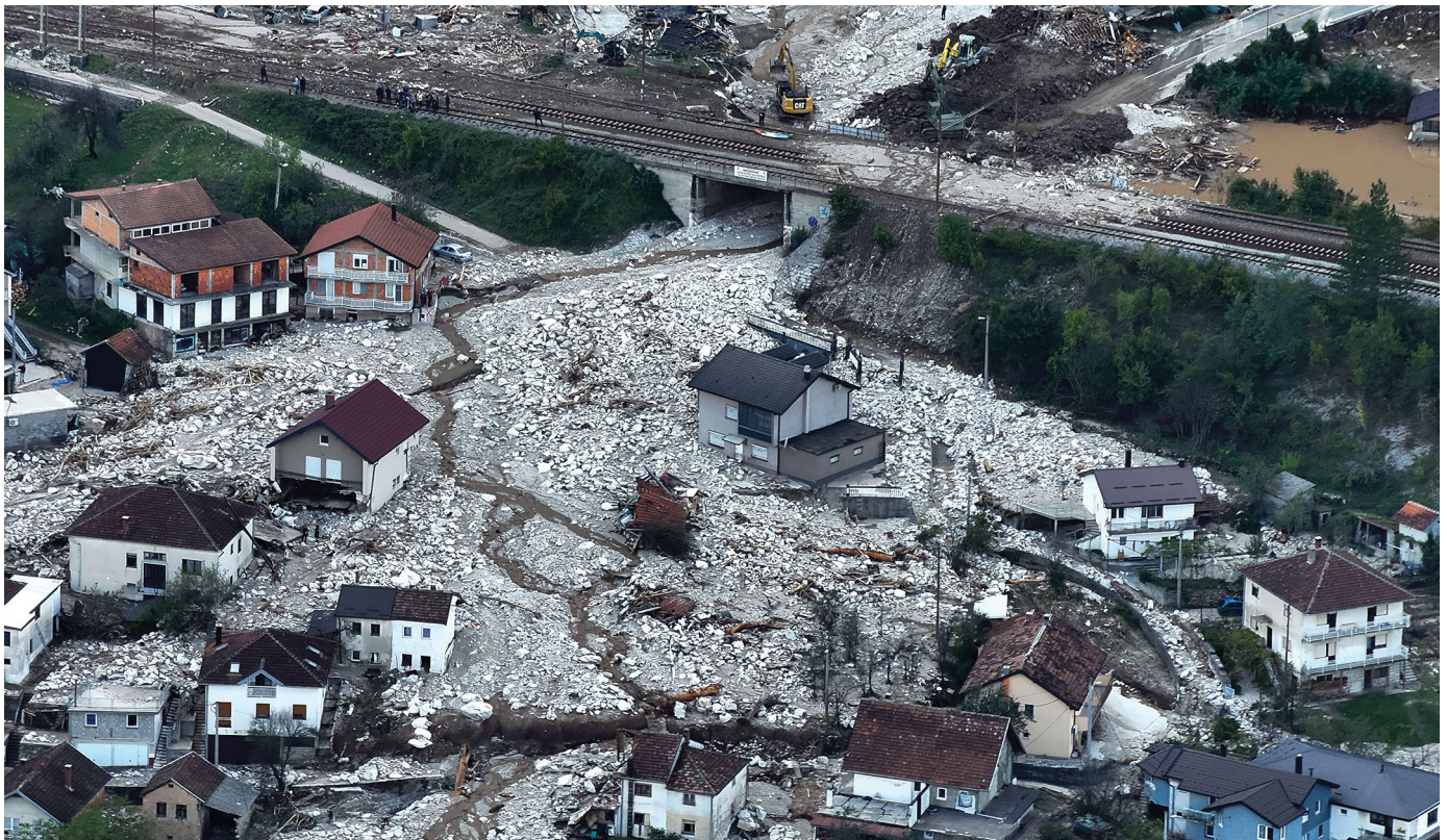
Figure 1: Flash floods and landslides in Donja Jablanica, 2024. © Jasminko Ibrakovic / Alamy
