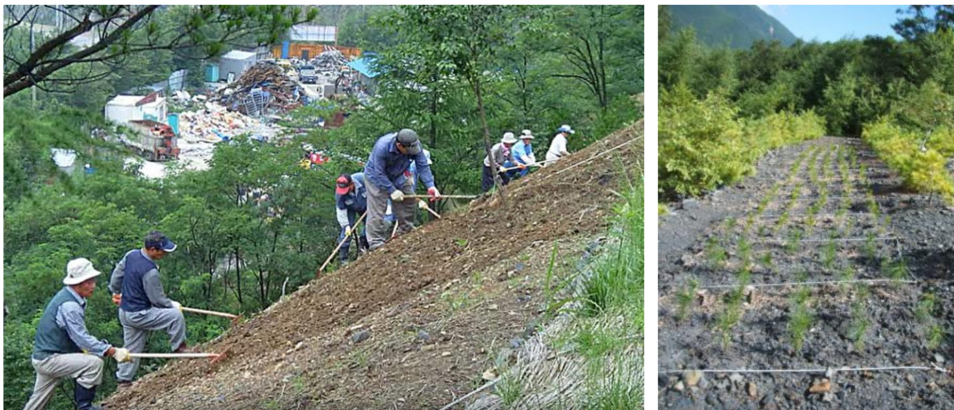
Figure 15 Left: slope grading of mine waste dump. Right: planting pine seedlings inoculated with Pisolithus for mine waste dump restoration.
