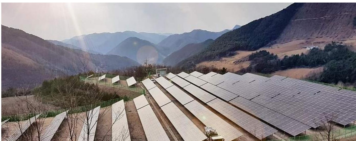
Figure 7 Solar Mine project on the waste rock pile from Hambaek mine.
