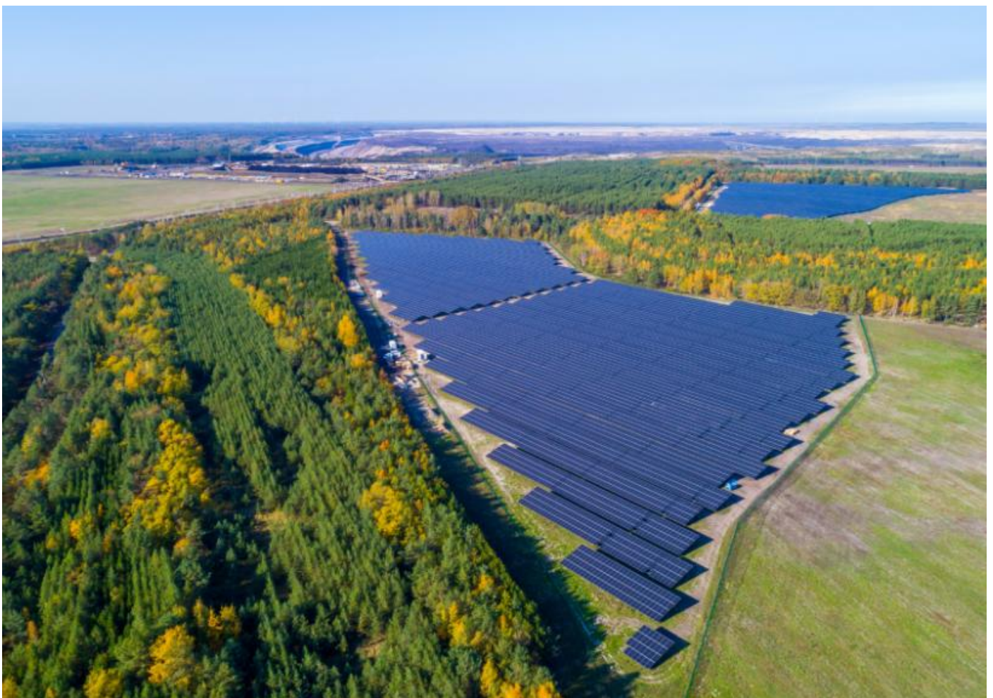
Figure 5 Haidemühl solar park on mining wasteland of the former Welzow-Süd mine.
