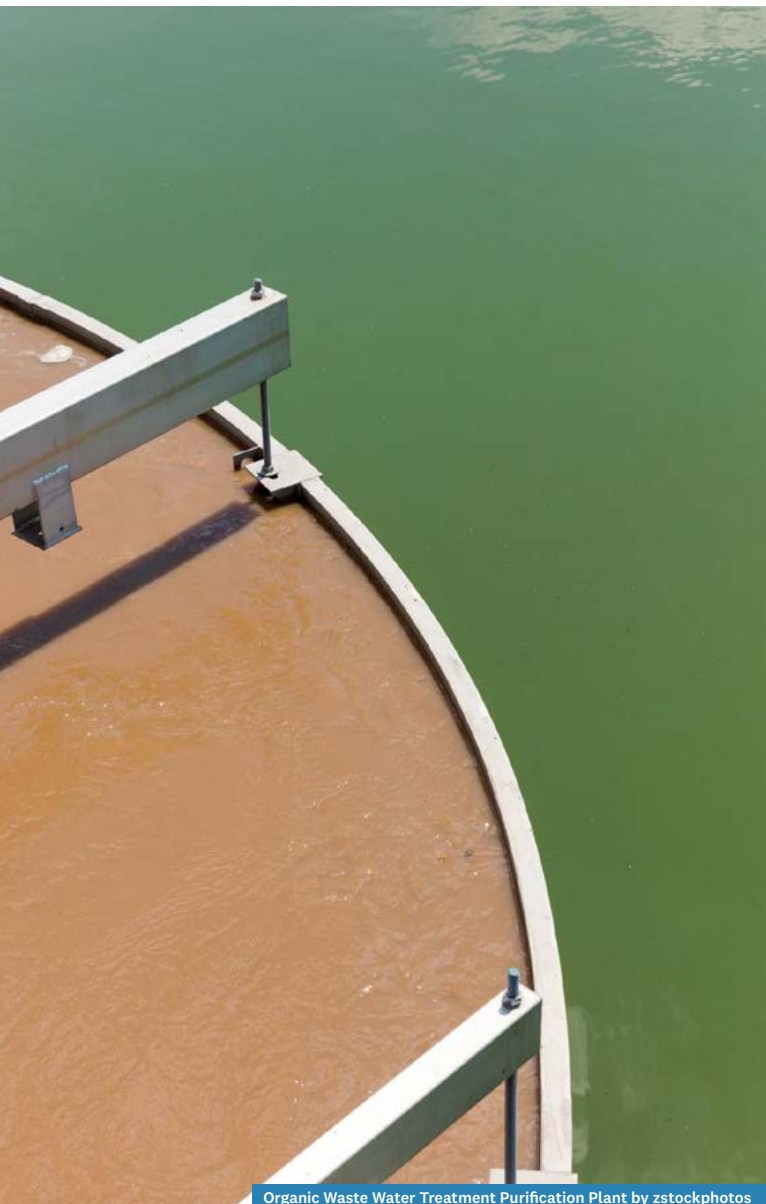
Organic Waste Water Treatment Purification Plant by zstockphotos
